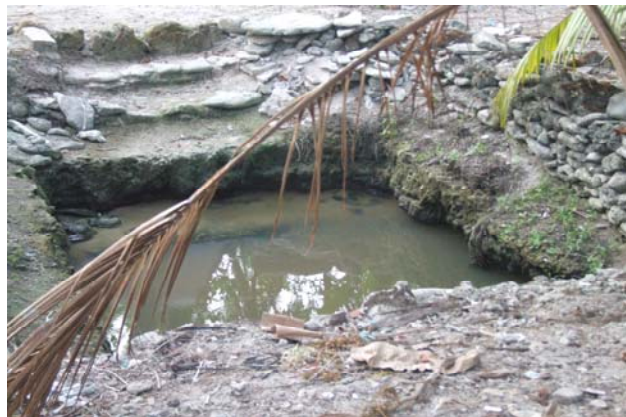
The traditional water body at Cheryam Satellite Island Proposes renovation under MGNREGS
