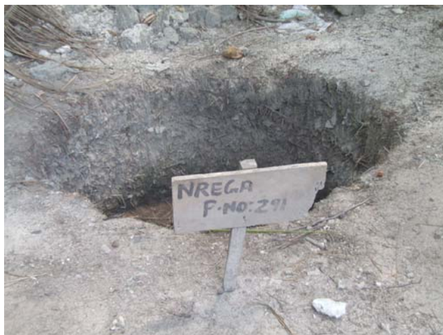
A well under construction at Andrott Island
